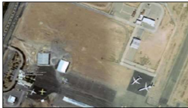
Figure 1. Aerial view of the cargo platform, cargo terminal (upper right), General Aviation (lower left), and hangars (lower center) of the Regional Airport under
